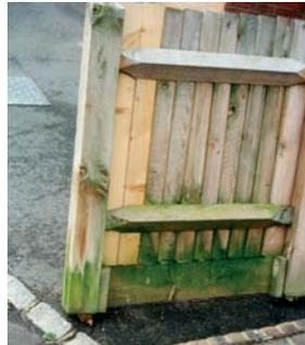
The reputation of timber for fencing is put at risk with bad practice like the photograph opposite – cross section reduced to fit a non-draining hole and no retreatment!
