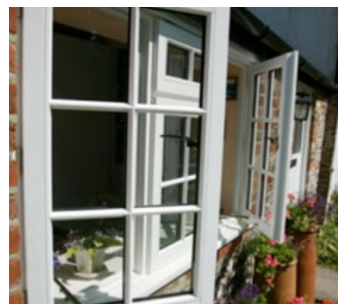
External timber joinery
