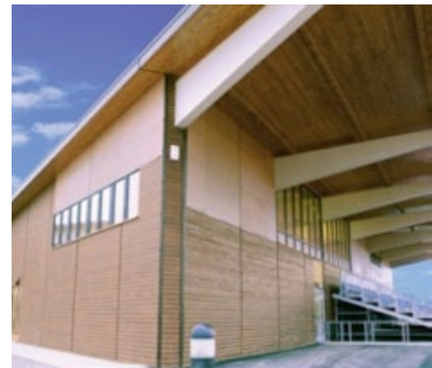
Boston Sports Stadium, Boston, Lincolnshire
