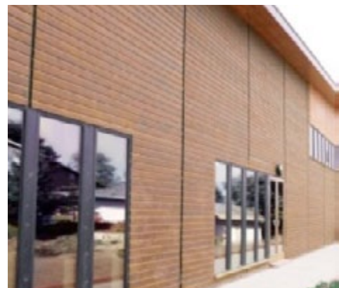
Boston Sports Stadium, Boston, Lincolnshire
