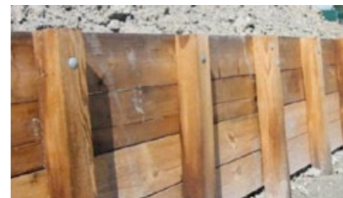
Retaining wall and piling
